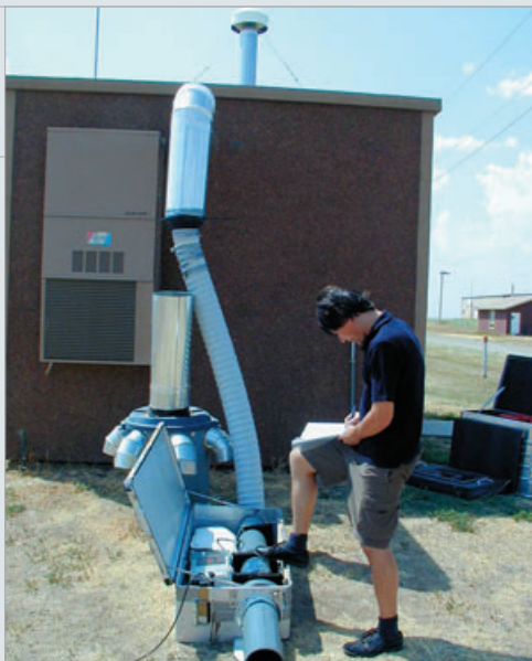
Airflow measurement check at radionuclide station RN74, Ashland, Kansas, USA.
