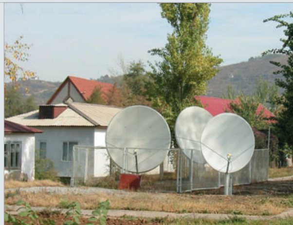
Primary seismic station PS23, Makanchi, Kazakhstan.
