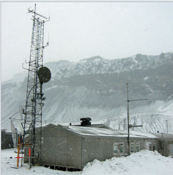
Auxiliary seismic station AS73, Jan Mayen, Norway.
