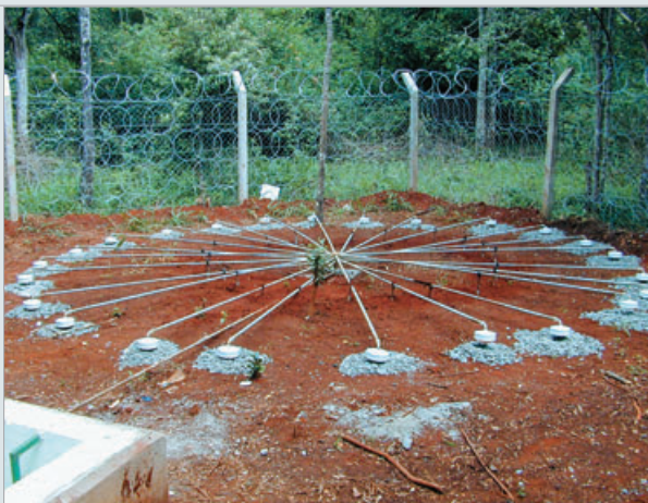
Wind noise reducing pipe array at infrasound station IS32, Nairobi, Kenya.
