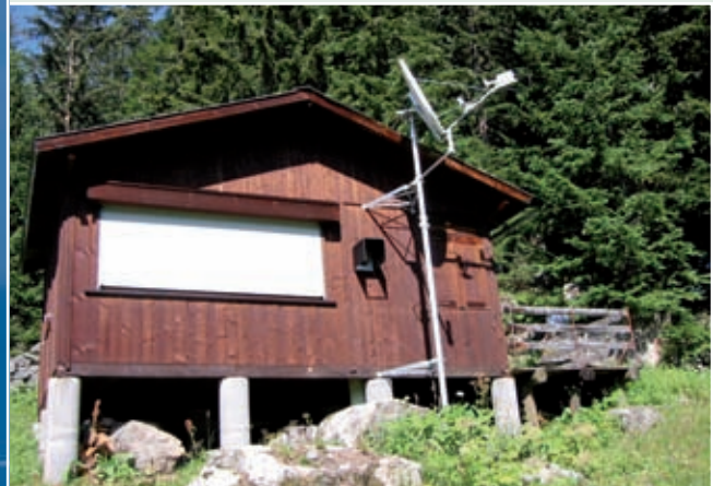
Auxiliary seismic station AS102, Davos, Switzerland.
