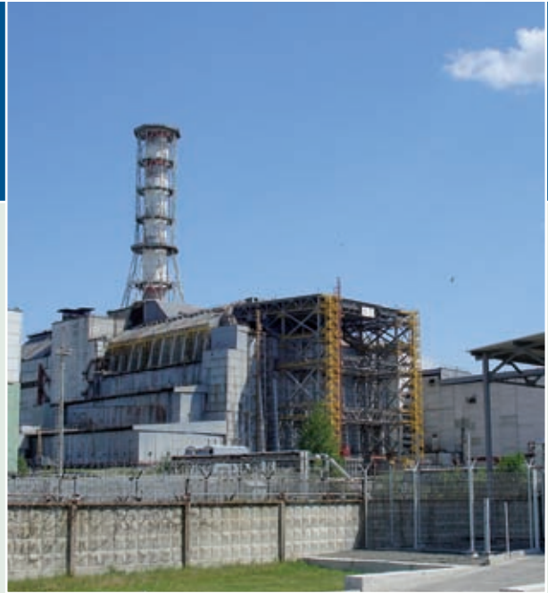
Concrete containment surrounding remains of nuclear power plant unit in the Chernobyl Exclusion Zone.
