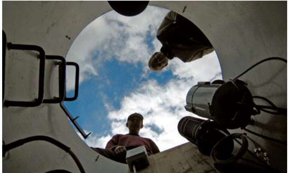
INSIDE AN IN-GROUND VAULT AT AN ASI04 ELEMENT, ESKDALEMUIR, SCOTLAND.
